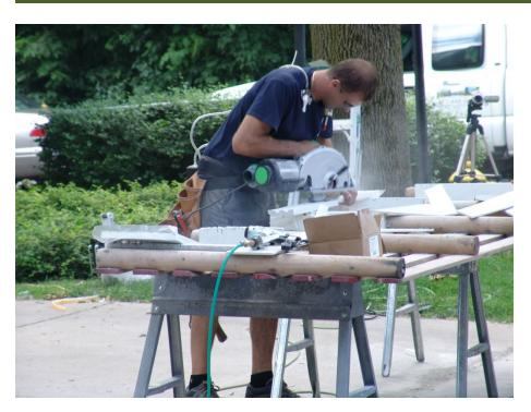
Figure 3 – A worker (cutter) cutting fiber-cement siding using a prototype circular saw with a built-in cyclone dust collector and an air filter ("red-spur saw"). Photo courtesy of NIOSH.
