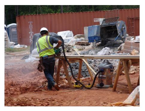
Figure 2 – A worker (cutter) cutting fiber-cement siding using a dust-collecting circular saw that was connected to a shop vacuum.
