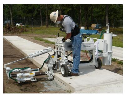
Figure 1 – Laborer Operating Dowel Drill
