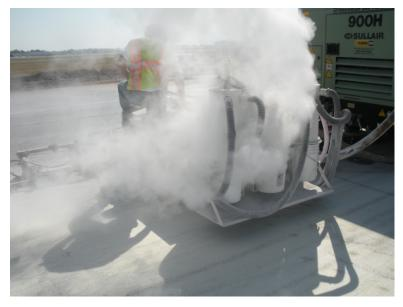
Figure 9 - Purging Creates Clouds of Dust
