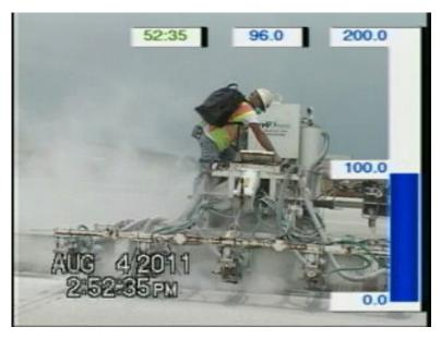
Figure 11 - Purging the Dust Collection System Produced a Spike in Respirable Dust Exposure
