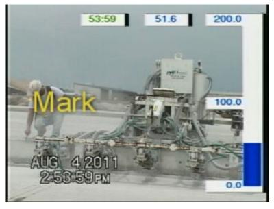
Figure 10 - Marking the Concrete During Drilling Produced a Spike in Respirable Dust Exposure
