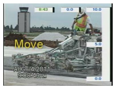
Figure 12 - Moving the Drill Did Not Result in a Spike in Respirable Dust Exposure
