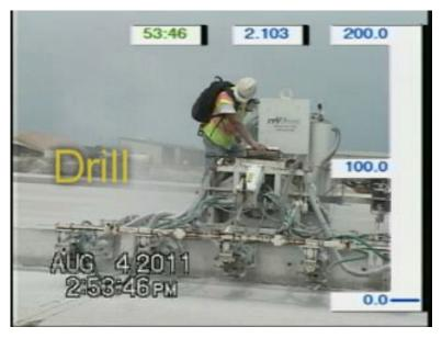
Figure 13 - The Drilling Task Did Not Result in a Spike in Respirable Dust Exposure
