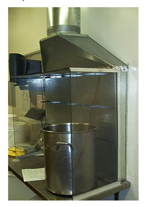
Figure 3. Ventilated booth-type exhaust hood.
