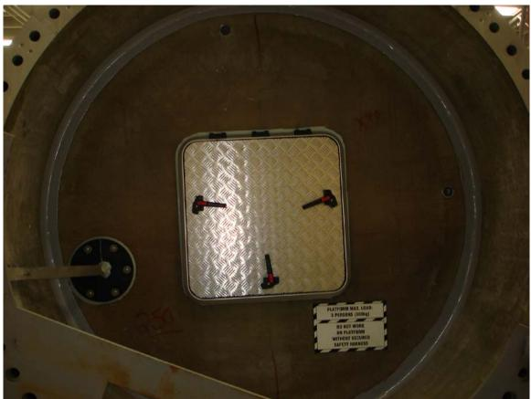
Figure 6: Installation of the chequer plate using Sika Flex.
