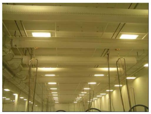
Figure 3: General ventilation supply in the M Building web cut and trim area
