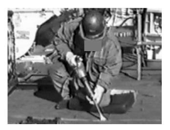
Figure 8. Worker Using Chipping Hammer to Remove Terrazzo Tile from Deck Surface
