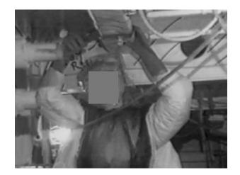
Figure 4. Insulation Worker Cutting into Insulation with Hawksbill Knife
