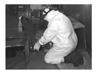
Figure 7. Worker Using Reciprocating Saw While Kneeling
