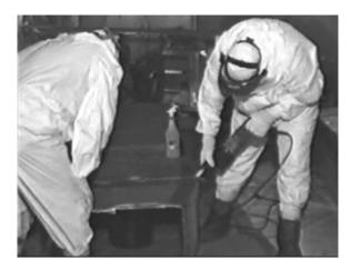
Figure 6. Two-Person Cutting Operation for Ductwork with Possible Hazardous Material
