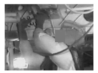
Figure 3. Worker Removing Insulation Tie Cap with Short Pry Bar
