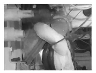
Figure 5. Pulling Section of Insulation Off Bulkhead by Hand
