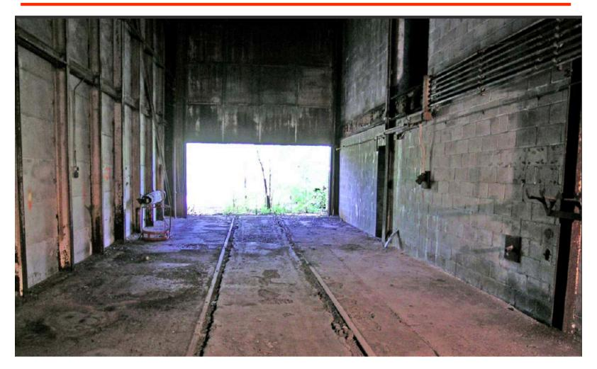
**LEGEND.** View from the Old Betatron railroad track tunnel looking out. Photo by Dan McKeel 2006. Double leaf metal door has exposed vertical struts that are not covered by lead shields. Workers confirm no lead shield.
