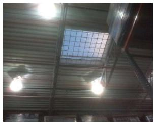
Figure 2 – Skylight guard with strengthening
