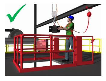
**Solution:** Encourage workers to use a personal fall arrest system when working near the opening of any unguarded area. Having only one side of an opening accessible with a safety gate and providing barriers on all other sides can further prevent falls through the opening.
