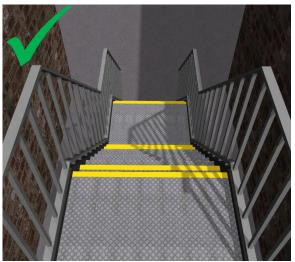
**Solution:** Clearly mark and highlight the edge of the stairs (nosing) using caution yellow or other high-contrast paint to increase the visibility of the nosing.
