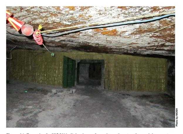
Figure A1. Example of a MICON built-in-place refuge alternative stopping and door system.
