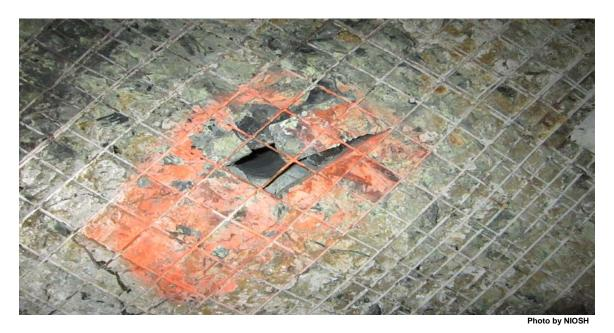
Figure A7. Breathable air supply borehole opening into a built-in-place refuge alternative with no collar.
