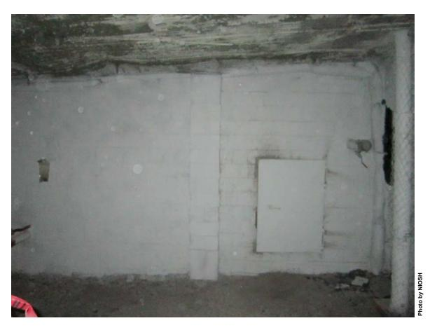
Figure A2. Mine-designed and MSHA District Manager-approved built-in-place refuge alternative stopping and door system.
