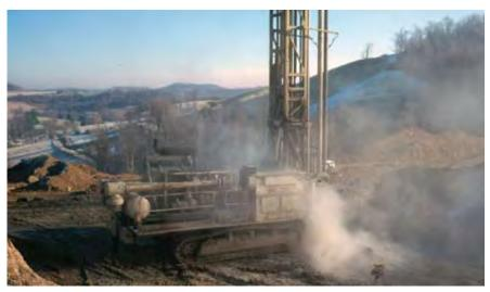
Figure 1. Rock drilling without appropriate dust control.
