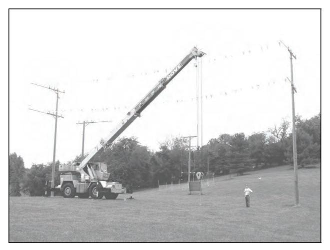
Figure 8.—Grove RT522 crane on outriggers, positioned adjacent to overhead power lines with boom at 50% extension and boom tip approximately level with lower set of lines.
