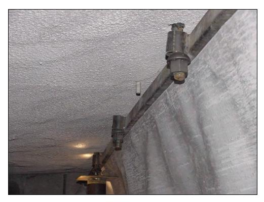
Figure 27.—Anchoring top box section to the mine roof.
