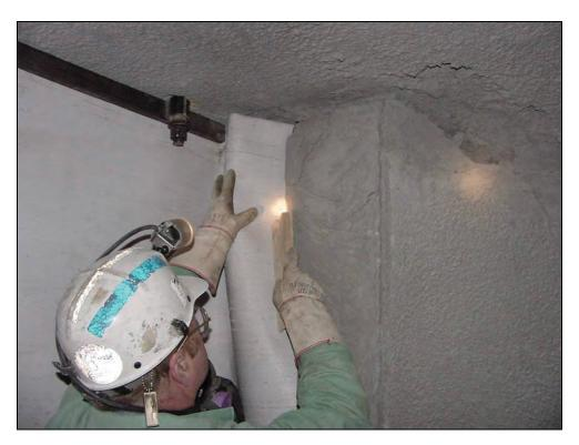
Figure 28.—Wedging woven cloth into mine rib.
