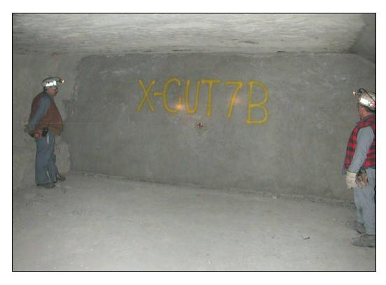
Figure 48.—The dry-stacked hollow-core concrete block stopping in X-7 remained intact after LLEM test #430.
