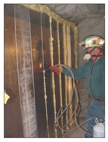
Figure 22.—Polyurethane sealant used on perimeter and vertical panel joints.
