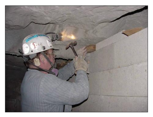
Figure 6.—Installation of wood header boards and wood wedges between the stopping and roof for dry-stacked hollow-core concrete block stopping.
