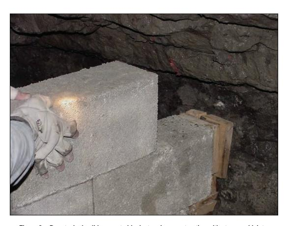
Figure 8.—Dry-stacked solid-concrete-block stopping construction with staggered joints.
