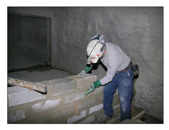
Figure 12.—Wet-laid solid-concrete-block stopping construction with staggered joints.
