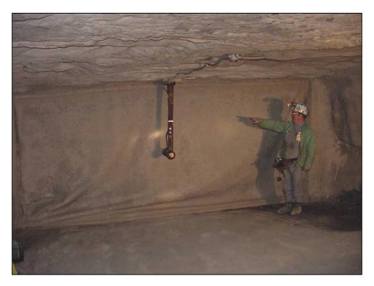
Figure 31.—Completed woven cloth stopping design in X-6, viewed from the explosion or C-drift side.
