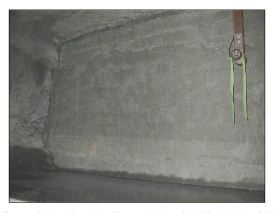
Figure 11.—Completed dry-stacked solid-concrete-block stopping in X-5 as viewed from C-drift, with the total explosion pressure transducer at the upper right.
