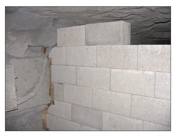
Figure 3.—Dry-stacked hollow-core concrete block stopping construction, with staggered joints.
