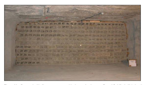
Figure 86.—Dry-stacked hollow-core concrete block stopping between B- and C-drifts in X-4 showing individually numbered block, viewed from C-drift.
