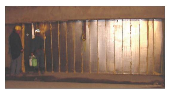
Figure 23.—Nearly completed steel panel stopping in X-6 showing closed, smooth panel sides facing C-drift.
