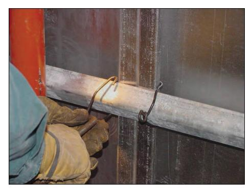
Figure 19.—Metal twist clamp used to secure open side of panel to the horizontal angle.
