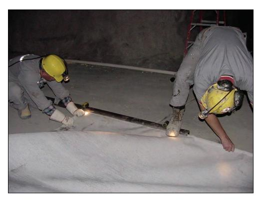
Figure 26.—Inserting pipe/sleeve into top box section.
