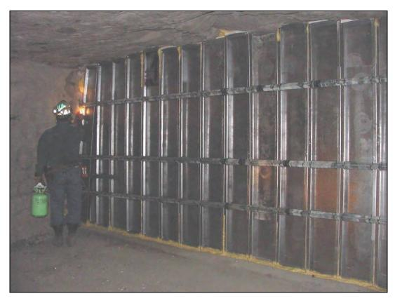
Figure 24.—Nearly completed steel panel stopping in X-6 showing the open panel side attached to the horizontal rib-to-rib angles on the B-drift side.
