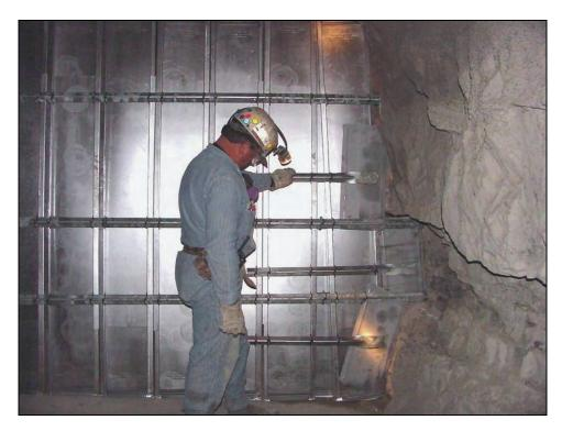
Figure 21.—Side extensions used to fill gaps between rib panel and rib, viewed from the back or B-drift side.
