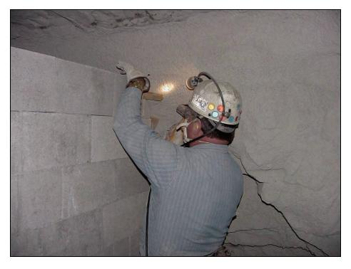
Figure 5.—Installation of wood wedges between the stopping and rib for dry-stacked hollow-core concrete block stopping.
