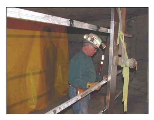
Figure 14.—Horizontal steel angles for attaching the steel stopping panels. The photo also shows the installed center panel.
