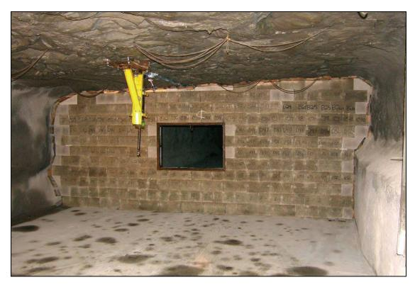
Figure 85.—Completed dry-stacked hollow-core concrete block stopping with simulated open regulator across B-drift.
