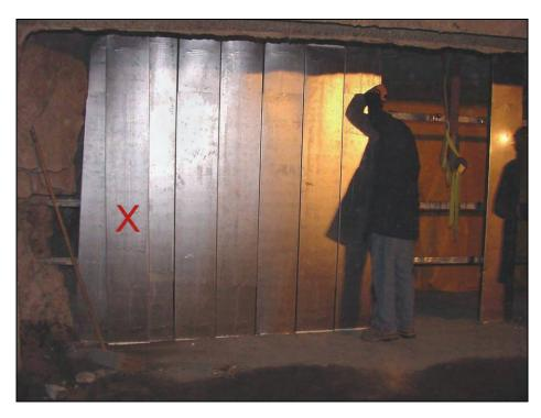
Figure 20.—Overlap panel (indicated by an "X") used to close gap between rib panel and second panel, as viewed from the front or C-drift side.
