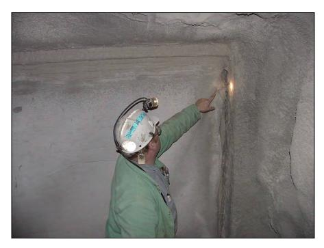
Figure 29.—Sealant along perimeter of the stopping, viewed from C-drift.
