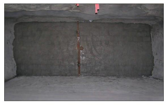
Figure 13.—Completed 6-in (15-cm) thick, wet-laid solid-concrete-block stopping in X-7, as viewed from A-drift.
