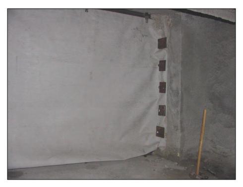
Figure 30.—Rib bolts installed in the X-6 stopping, viewed from B-drift.
