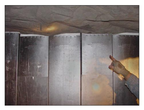
Figure 17.—Polystyrene foam head seal used to provide enhanced closure between metal panel and roof, as viewed from the C-drift side.
