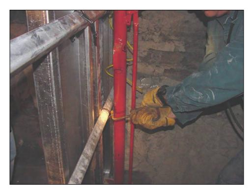
Figure 16.—Horizontal steel angles (with open sides facing panels on left), as viewed from B-drift.
