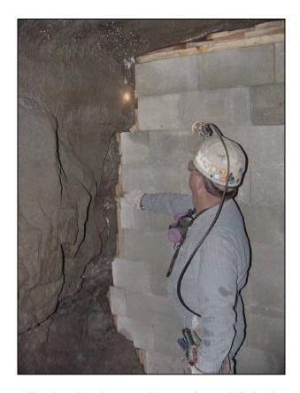
Figure 9.—Wood wedges between the stopping and rib for dry-stacked solid-concrete-block stopping.
