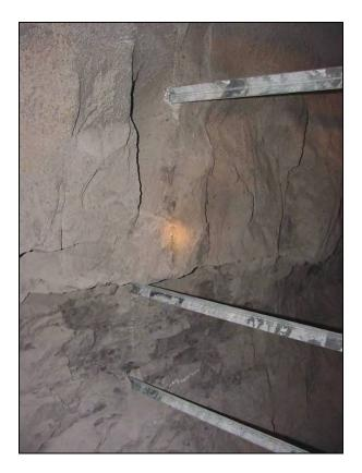
Figure 15.—Three horizontal steel angles inset into rib.
