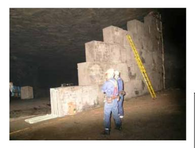
Figure 2.—Partially constructed Super Stopping.
