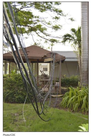
\* The cables shown directly powered a section of the laboratory's facility and were knocked down by the storm.
